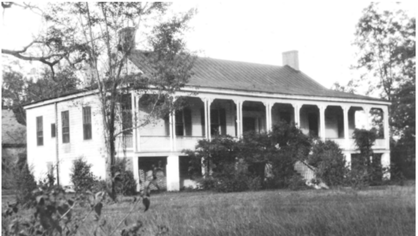
The T. L. Toulmin house in Toulminville, before the move and restoration
